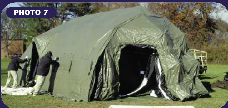
The interior bladder is inflated by a small, portable blower to raise the shelter.
